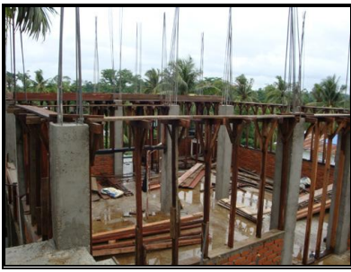
The beams for the third story of the new KBC Healthcare Clinic building are being set in place as of May 23, 2009.
